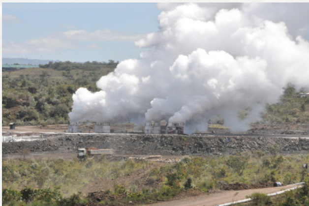
Wells of power... One of the geothermal wells at the Menengai Geothermal Project
